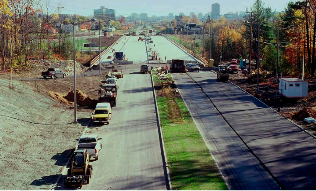
Boulevard des Allumettières under construction, Fall 2007. Photo: Doug Anions
